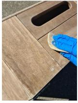
1) Wearing gloves, apply the oil liberally with a rag or large paintbrush. Rub excess off with a clean rag after 1-2 mins ensuring to wipe along the grain.
