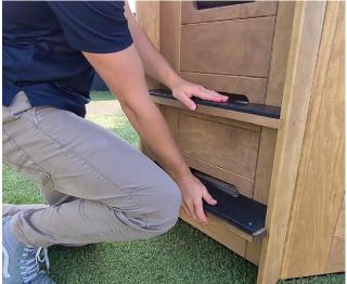
A3.5 The Overhead Branch climber can be mounted to any of the 3 equal sides of the Trapezoidal climbers. Do not mount it on the long edge as it will only allow for one fixing point. (Shown below)
